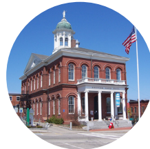
4 SAA AT TOWN HALL 10 Front Street *Exhibit on second floor
